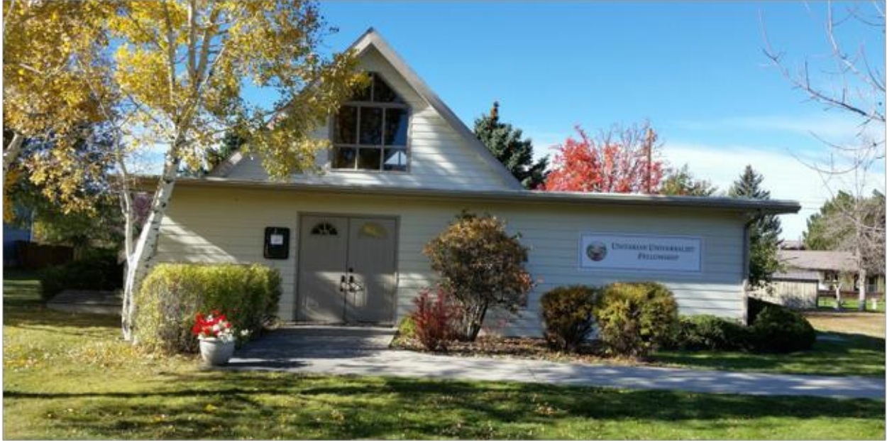
The Unitarian Universalist Fellowship of Bozeman’s building as it was prior to our renovations.
